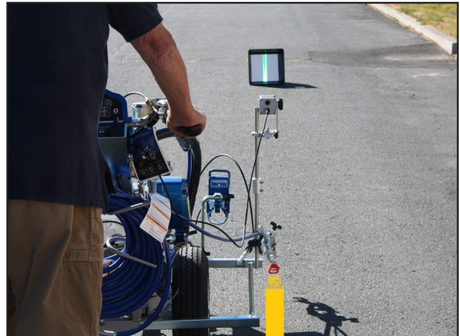
LaserLine's tool for walk behind paint striping machines allows for painting lines over 500 feet long.
